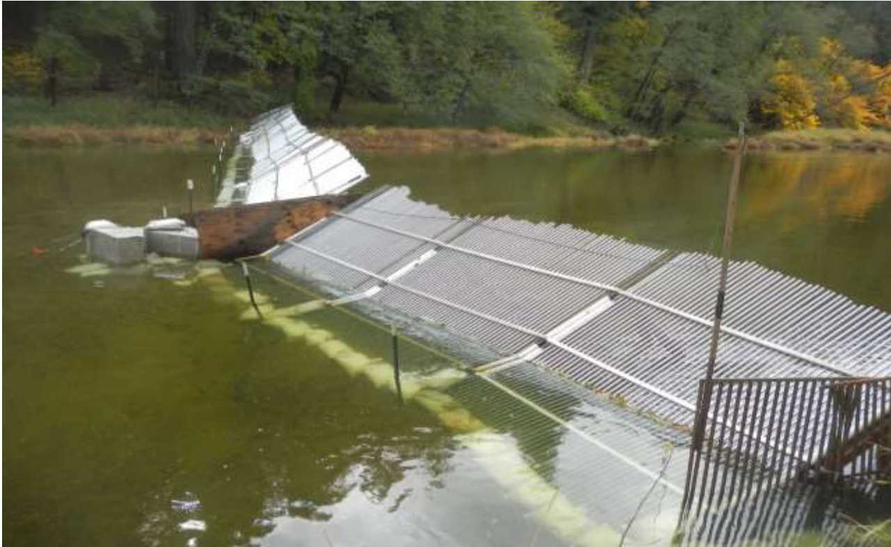
Figure 3. Scott River Fish Counting Facility located in Siskiyou County, California 2020.
