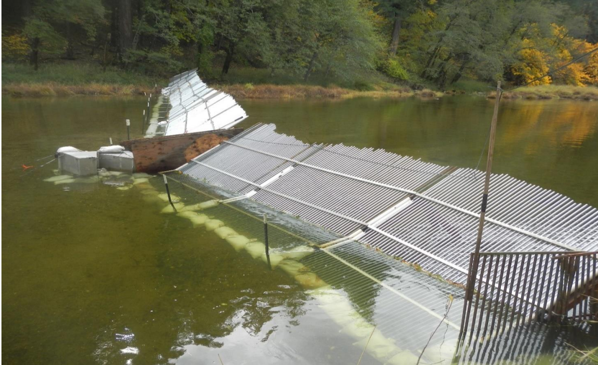
Figure 3. Scott River Fish Counting Facility located in Siskiyou County, California 2022.
